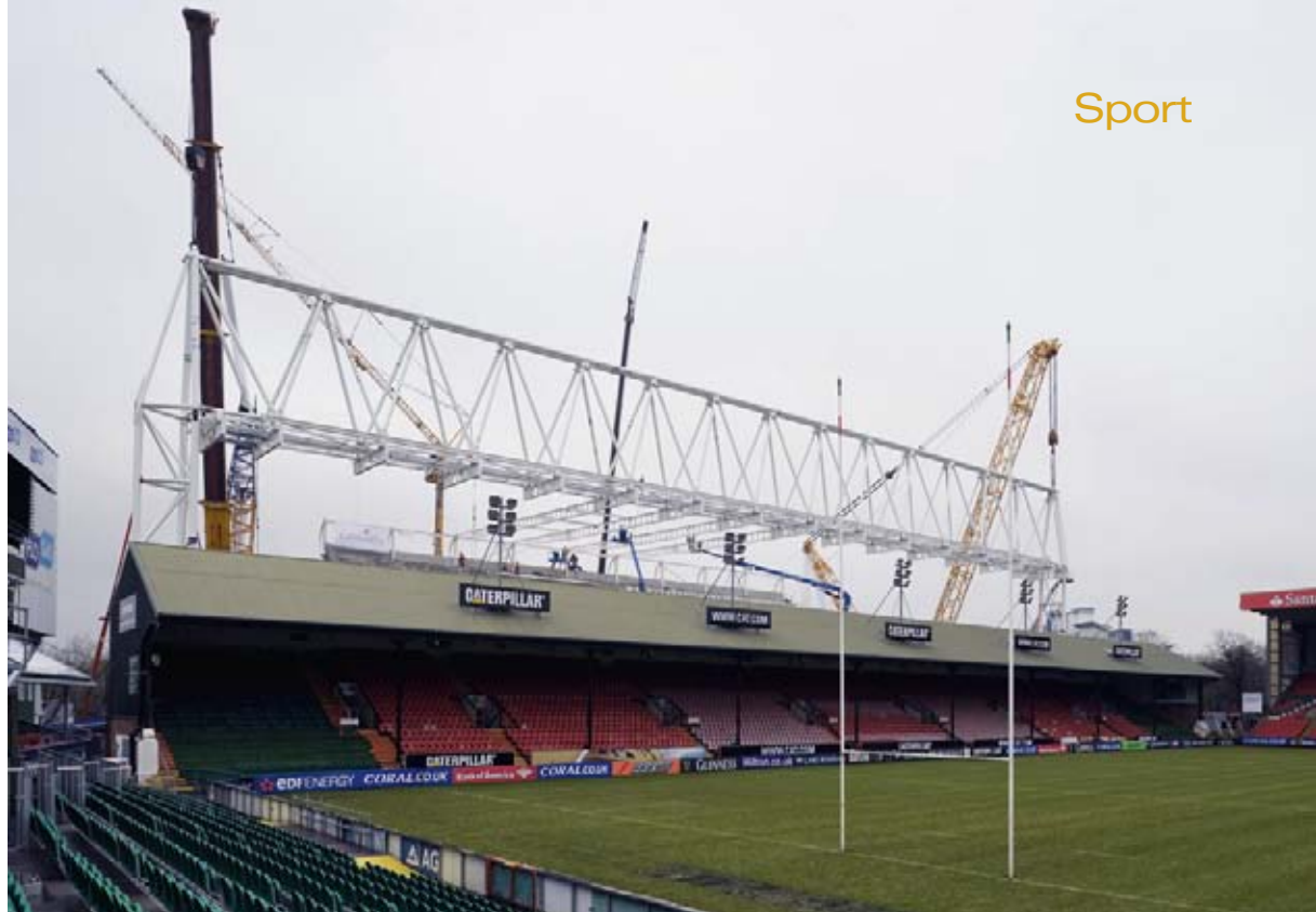
Above: The roof's truss was lifted into place in a dual lift by two 1,000t capacity cranes.
