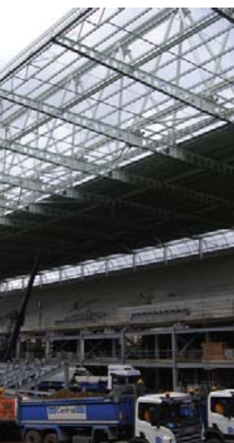
Below: Cellular beams in three sections form the stand's cantilever.
