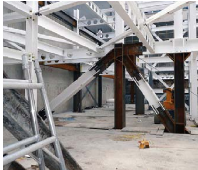
Above: A vierendeel truss was erected to cantilever over subterranean obstructions.
