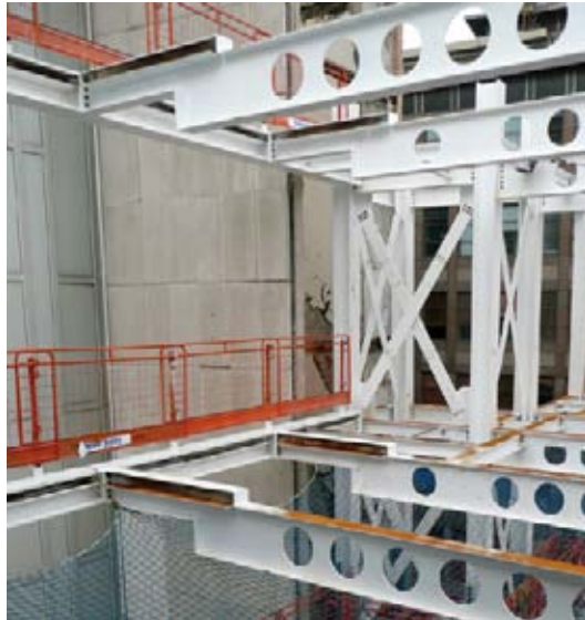
Above: The crank detail of the cellular beams which provides the thin floor level.
