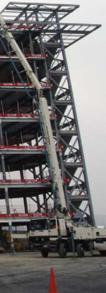
Above: Bracing has been positioned in lift shafts and partition walls.
