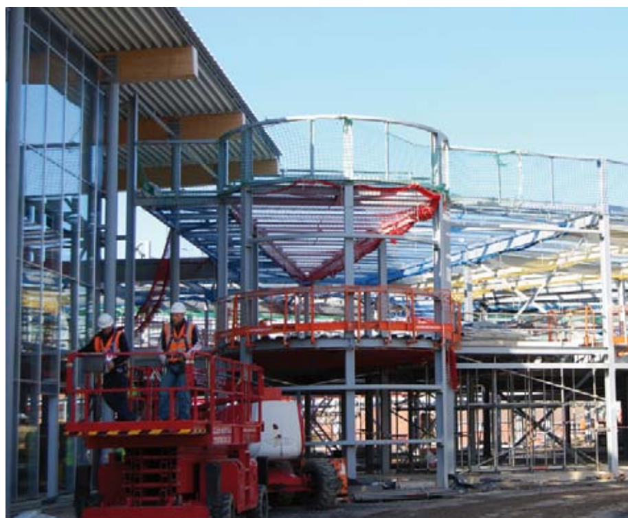
Below: The curved frontage of the school's entrance block.
