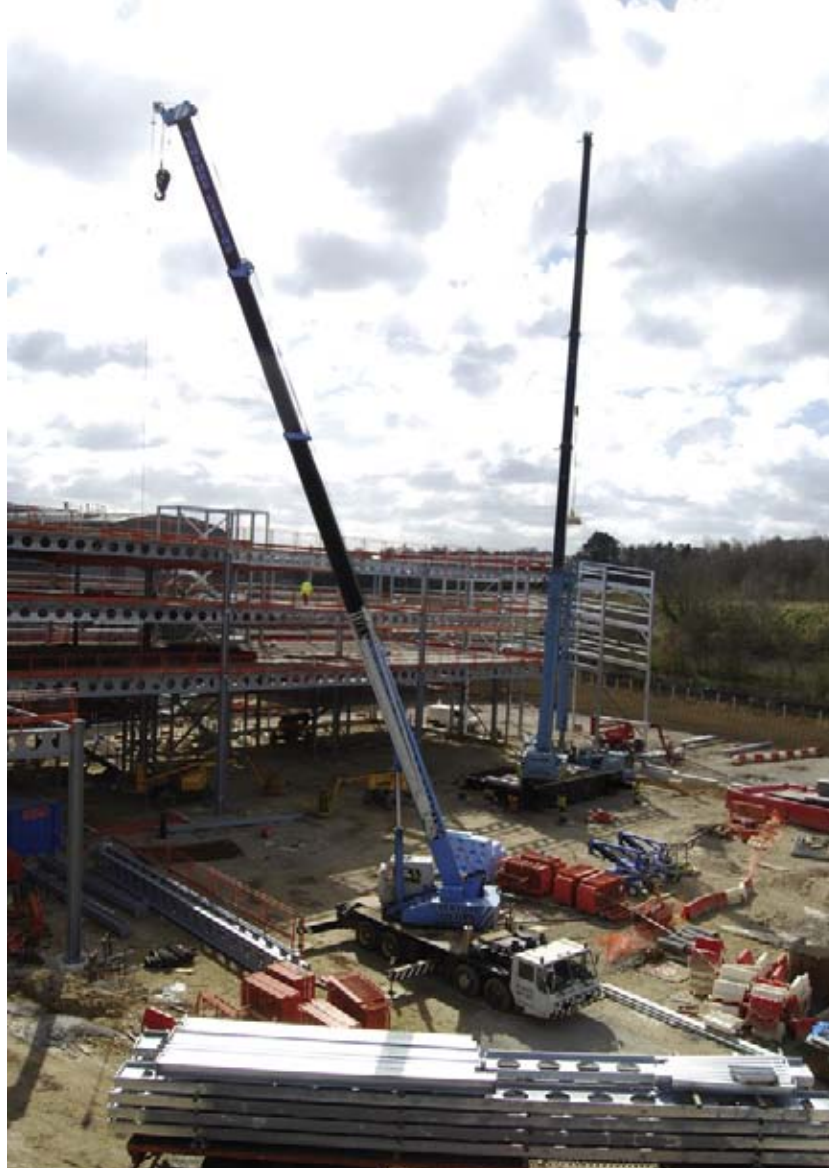
Left: Barrett Steel has installed both steelwork and concrete planks.
