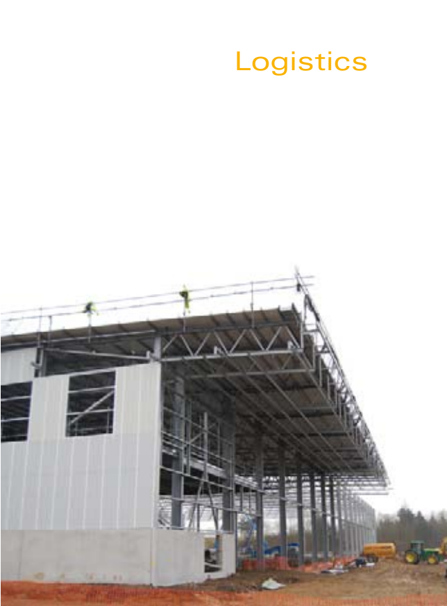
Above: A steel overhang protects the building's loading bays.
