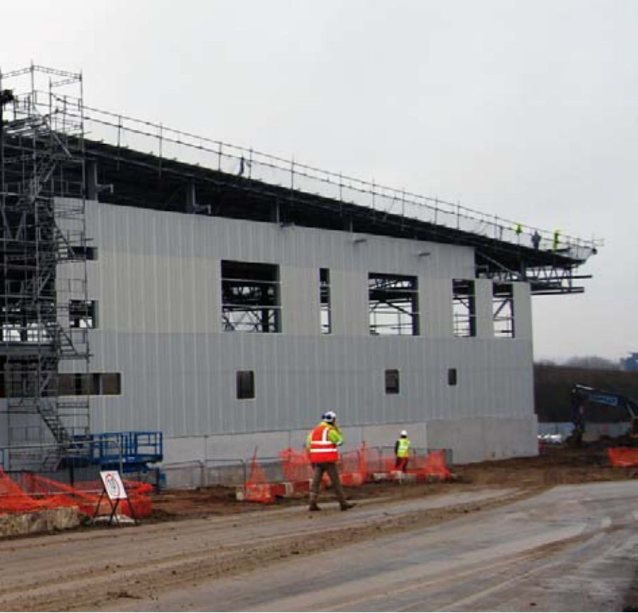
Above: The building's rear elevation features a two storey office block.
