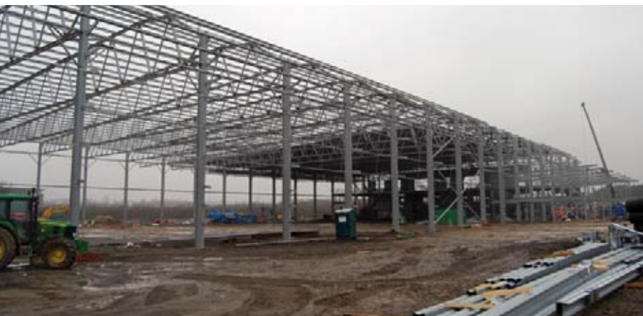
A series of 60m long trusses form the open column-free zone.
