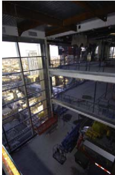
Far left: Triple height windows light up the building's atria
